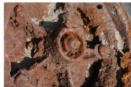
Figure 4: Pump erosion corrosion
