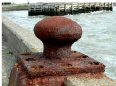
Figure 1: Bolted post showing uniform corrosion [13]
