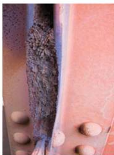
Figure 8: Pack Rust between steel plates [13]
