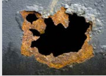
Pitting corrosion due to excessive chloride ion
